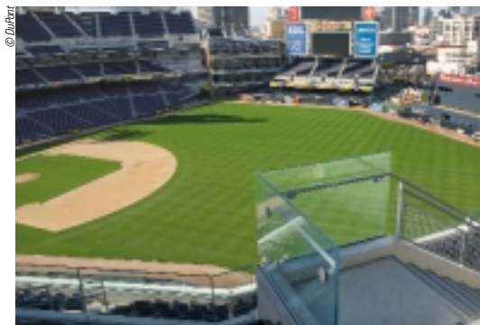
Sports fans worldwide can benefit from clear views thanks to balustrades of laminated glass using SentryGlas® Plus like these at the San Diego Padres' Petco Park ballpark.
