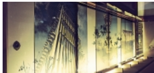
The temple's traditional paper doors were replaced by large panels of laminated safety glass containing photographs of the architect's work, made possible by SentryGlas® Expressions™ technology.
